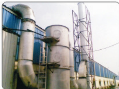
Fume Scrubbing System at Garg Inox, Pune (Acid Fumes)
