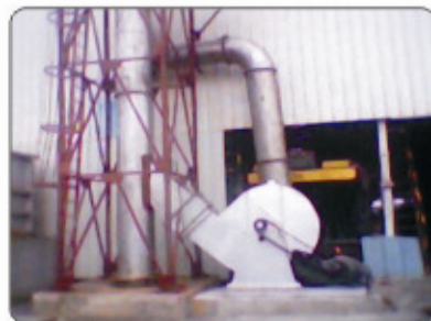
Fume Extraction System at Kalyani Thermal at Pune (Forging)
