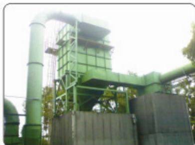
Dust Collection System at Tata Motors (Foundry): Bag Filter-262 Bags & Centrifugal Fan- 300H.P.
